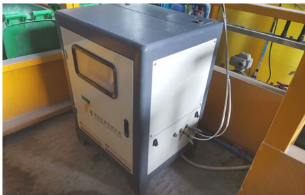
車間噴霧降溫裝置改善工作環境 Spray Cooling System Enhancing the Workshop Environment
